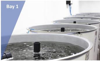
Eighteen (18) tanks in system (500 L each) with full RAS. The Bay can be operated for both feed or challenge trials. Freshwater or marine species system.
