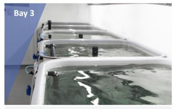
This bay has a dividing wall with two completely separate RAS units on each side. An interconnection is possible if required. The bay is currently used for quarantining and stock-holding of marine fish.
